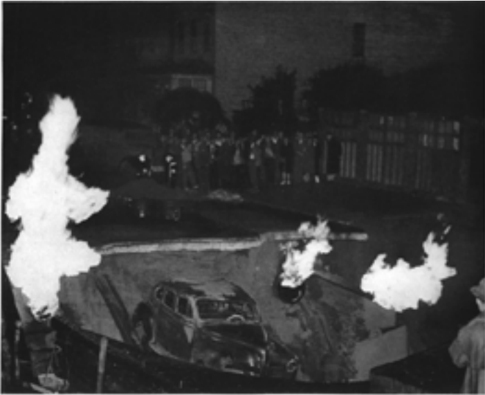
Mains Broke, Gas Burned, and a Car Fell into the Subway When a Bolt Struck in Brooklyn Gas lines under the street were supported by temporary decking. When lightning smashed the props, pipes collapsed and gas caught fire. Gas in tanks or subsurface mains cannot be exploded by lightning.
